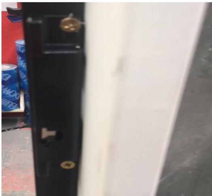
11. Fit the cover and install 2 x screws.
