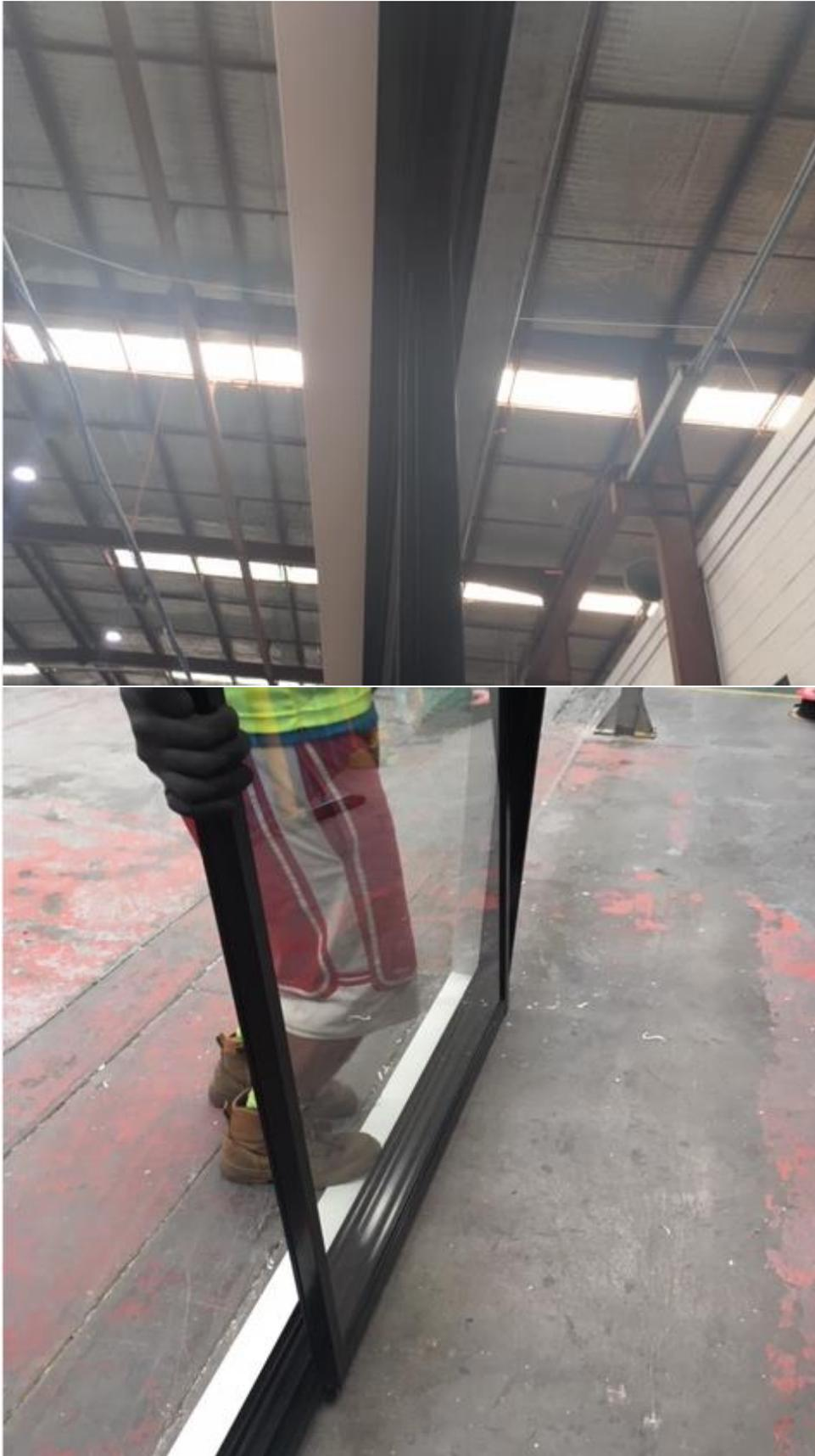
3. After installing the fixed panel, using the 3 x 8g x 13mm Gold zinc screw, screw the blocks into the head and sill making sure the panel is pushed all the way into the jamb.
